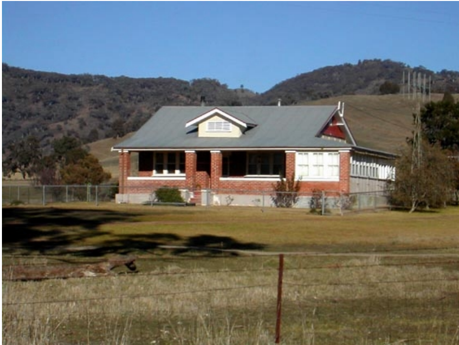
Photo 2.17: Conventional Housing on Rural Smallholdings Date of Photo: June 2002
