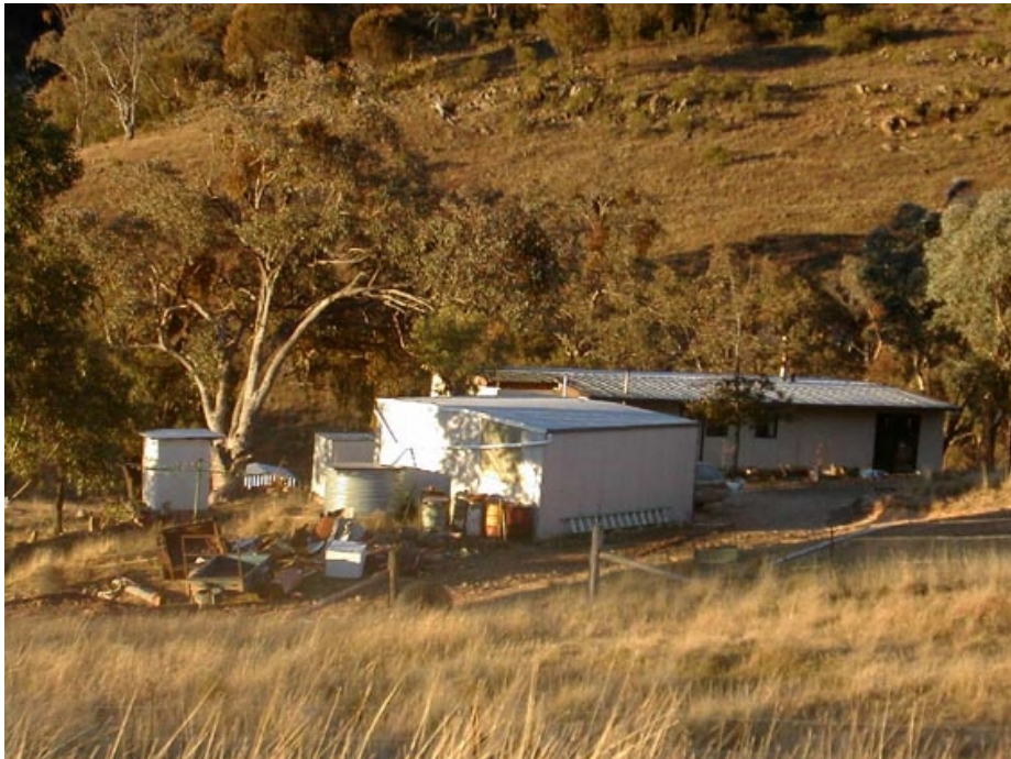
Photo 2.18: Rustic Housing on Rural Smallholdings Date of Photo: July 2002
