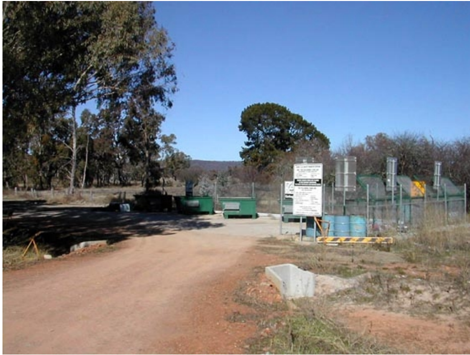
Photo 2.11: Waste Transfer Station at Kains Gap
