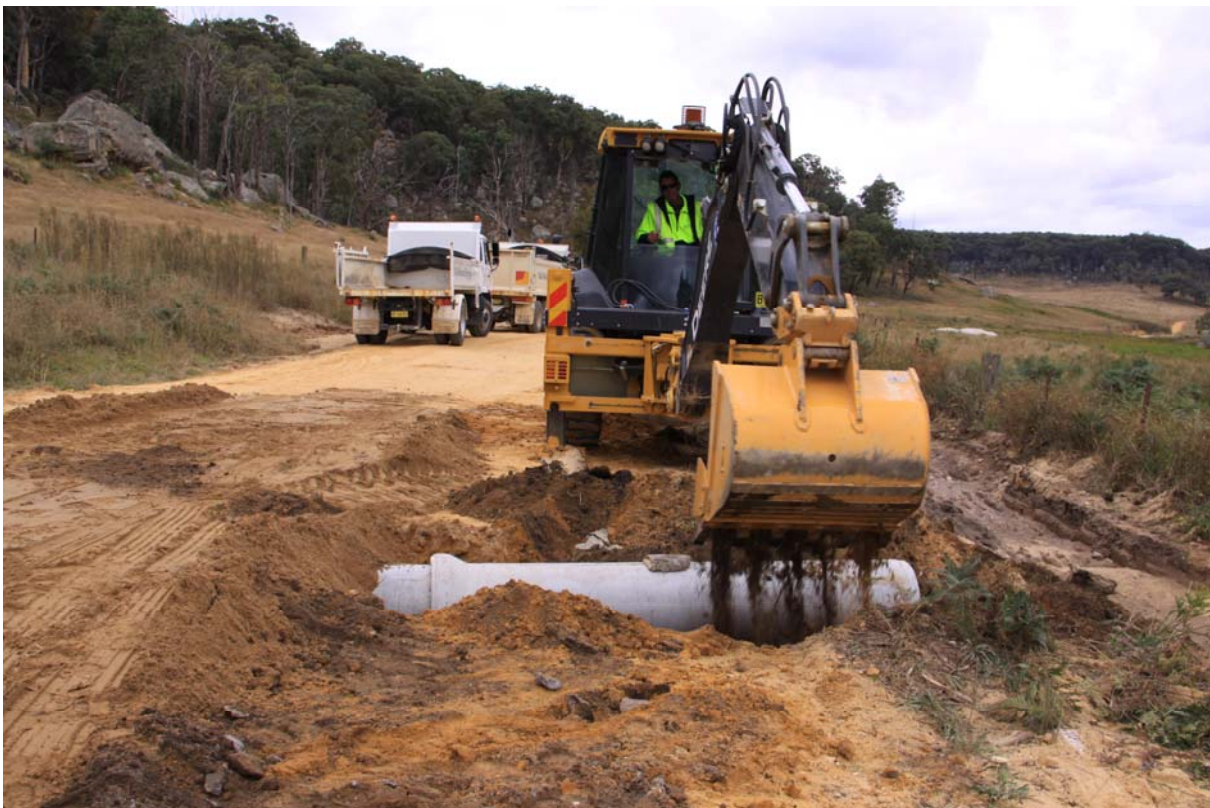
Installation of storm water pipe on Coricudgy Road
