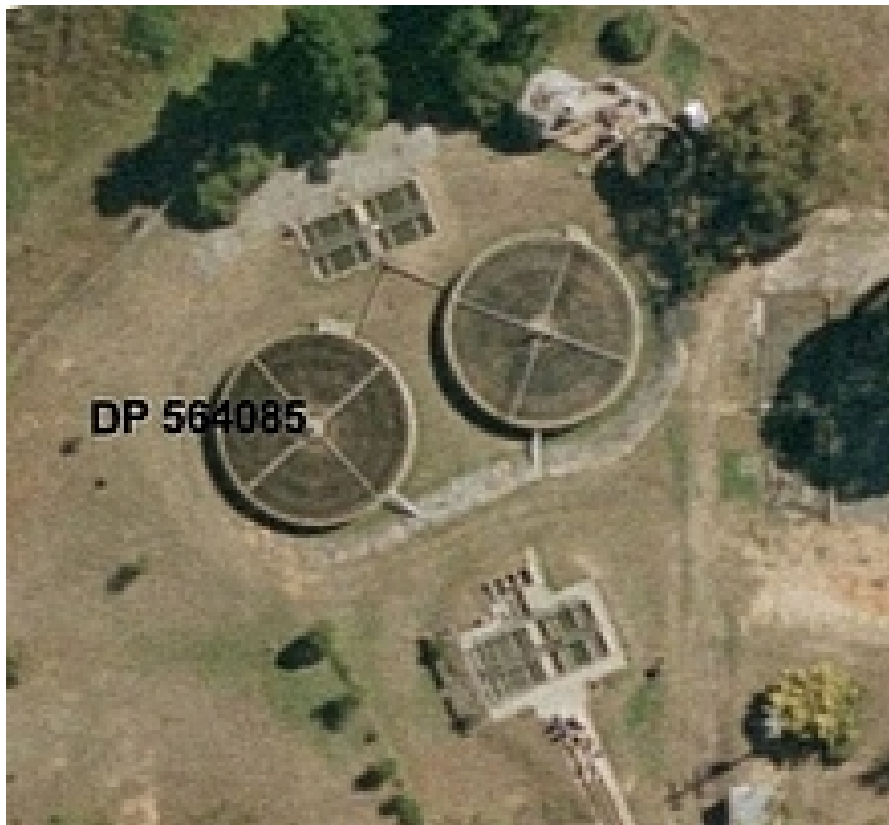
Existing Kandos sewer treatment plant
