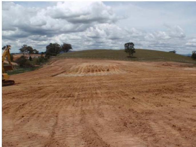
Photograph 4. The site stripped of topsoil
