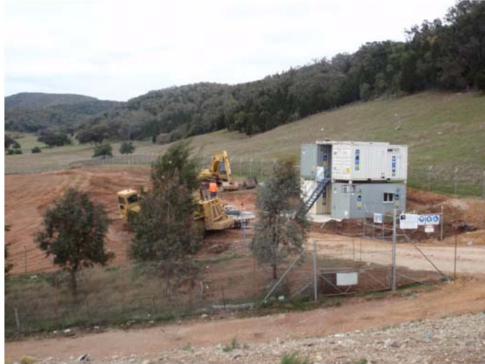
Photograph 1. PCI Site Office and Amenities
