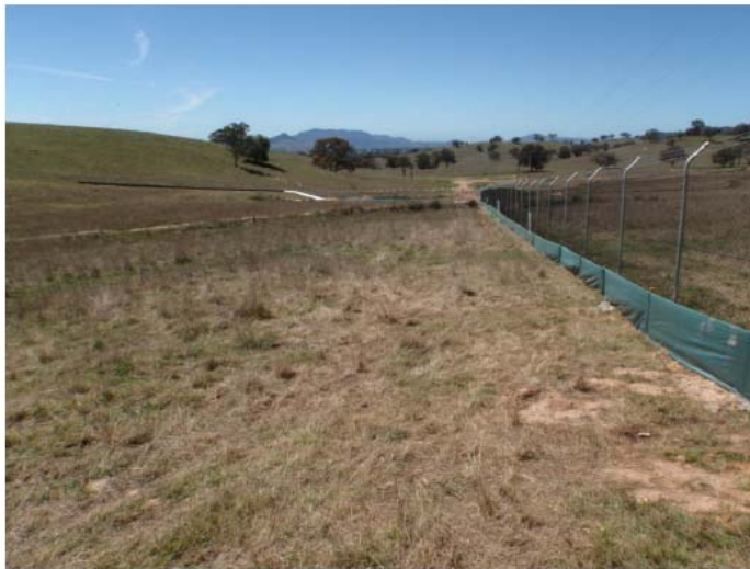
Photograph 2. Silt Fencing along the Southern Boundary
