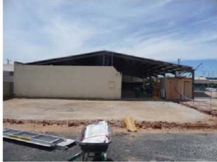
PROGRESS PHOTOS AS AT 28 NOV
