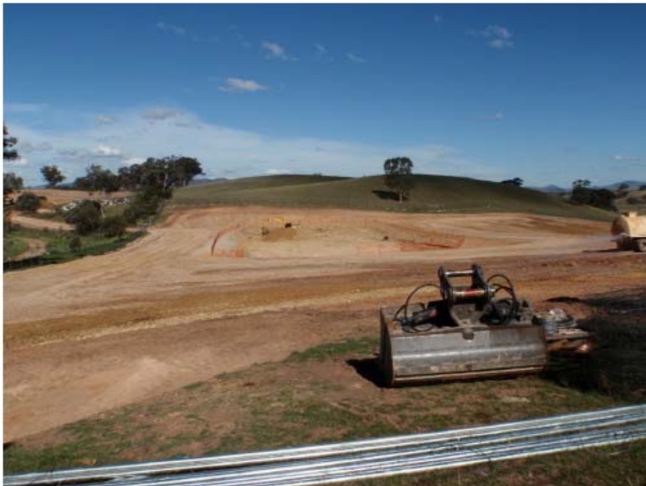
Photograph 1. Excavation for Aeration Tanks and road formation under construction.
