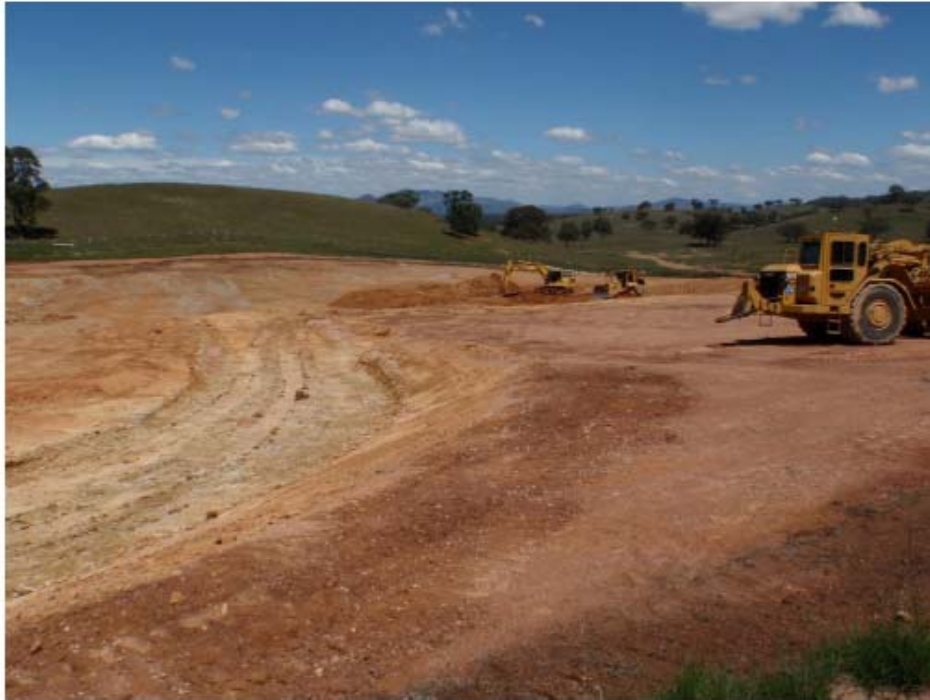
Photograph 2. Excavation for Sludge Lagoons and road formation under construction.
