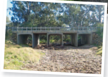
NEW BOX CULVERT BRIDGE
