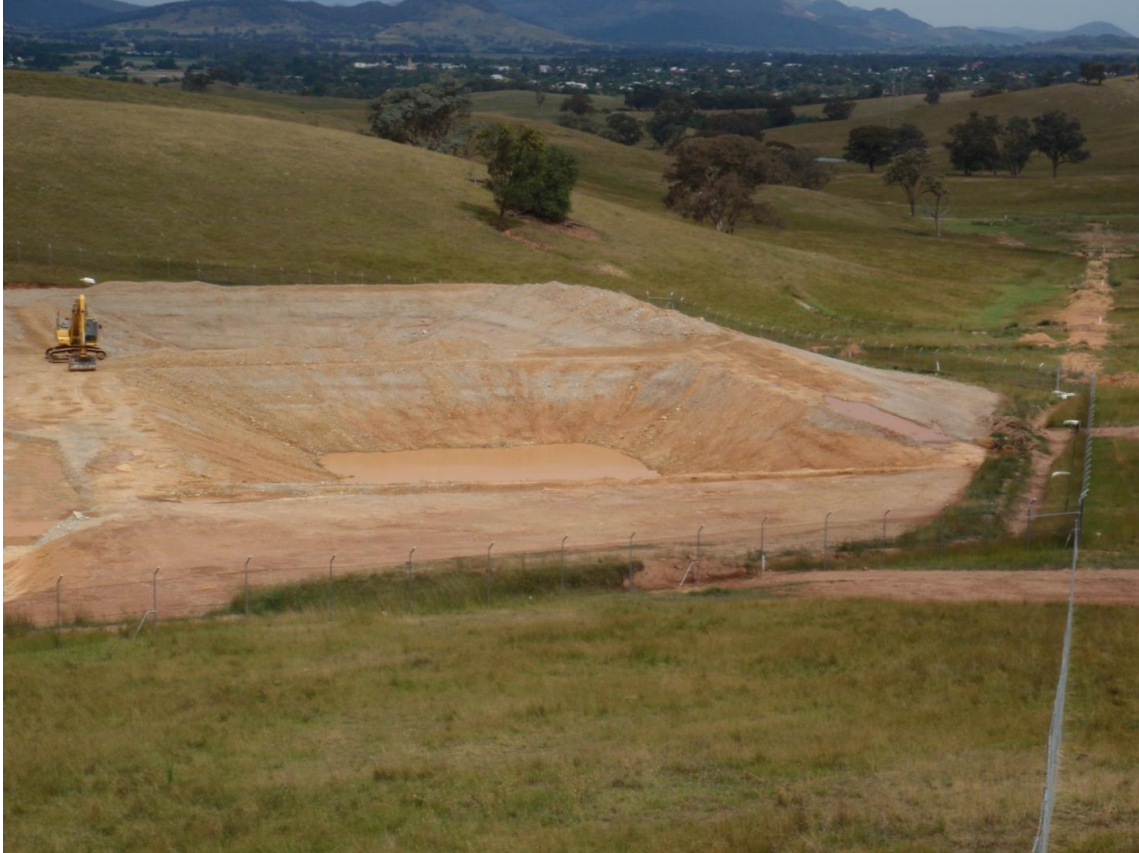
Photograph 2. Sludge Lagoons earthworks near completion.
