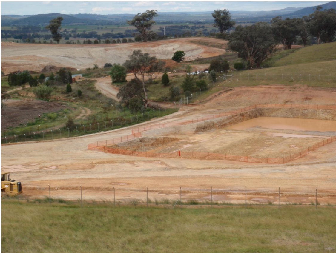
Photograph 1. Excavation for Aeration Tanks and Catch Balance Tank
