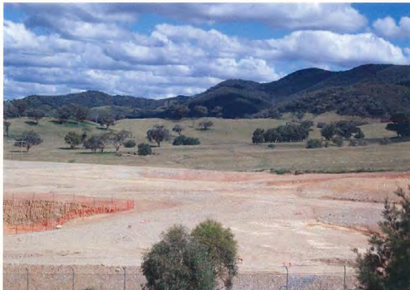
Photograph 1. Completed pads and set-out for administration building and inlet works structure.
