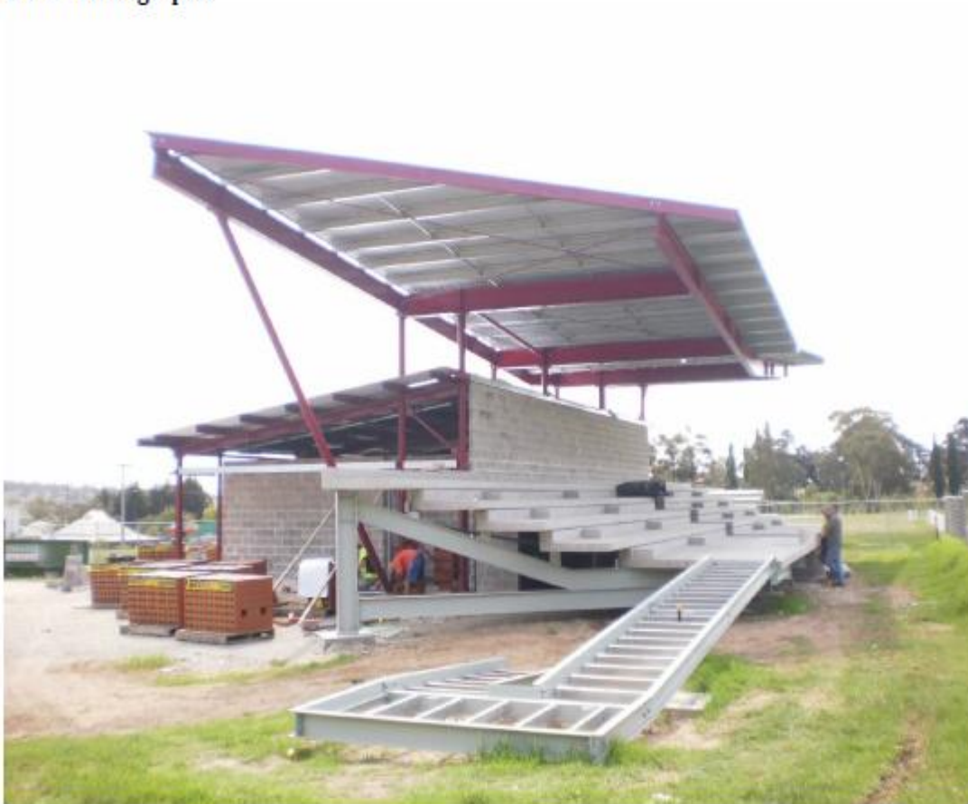
Photograph 1. Roof on, brick work nearing completion and plaths in place.
