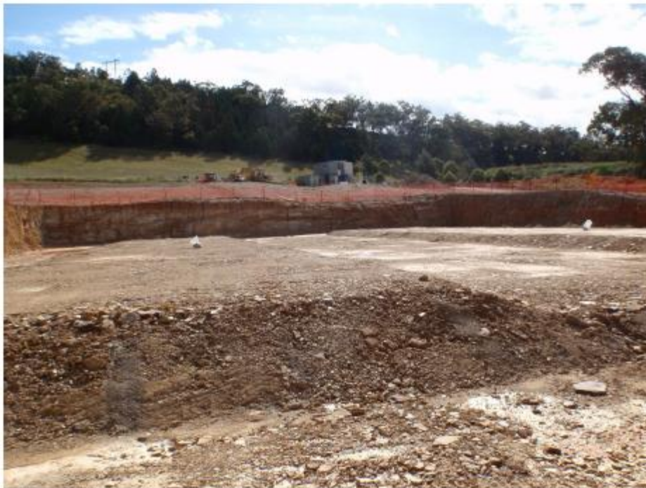
Photograph 1. IDEA Tank excavation prepared for concrete blinding layer.
