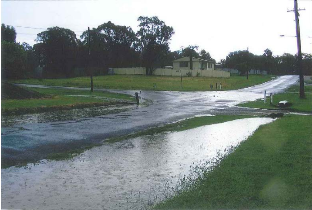
■ Figure 2-3 Stormwater impeded by culvert under the Driveway of 15 George Street
