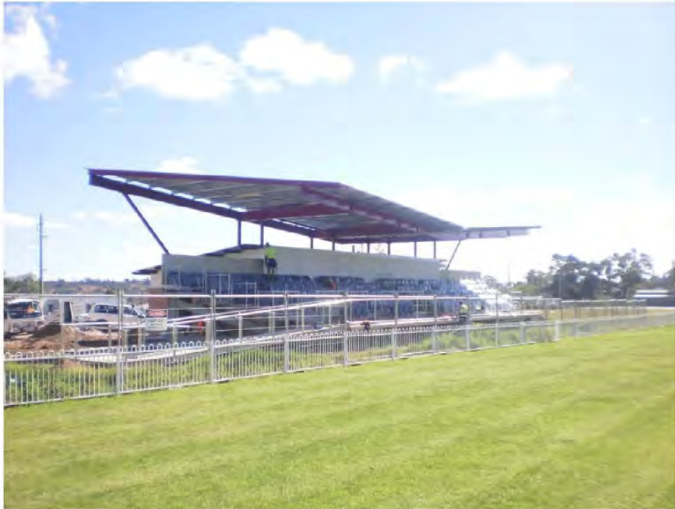
Photograph 1. Grandstand nearing completion.
