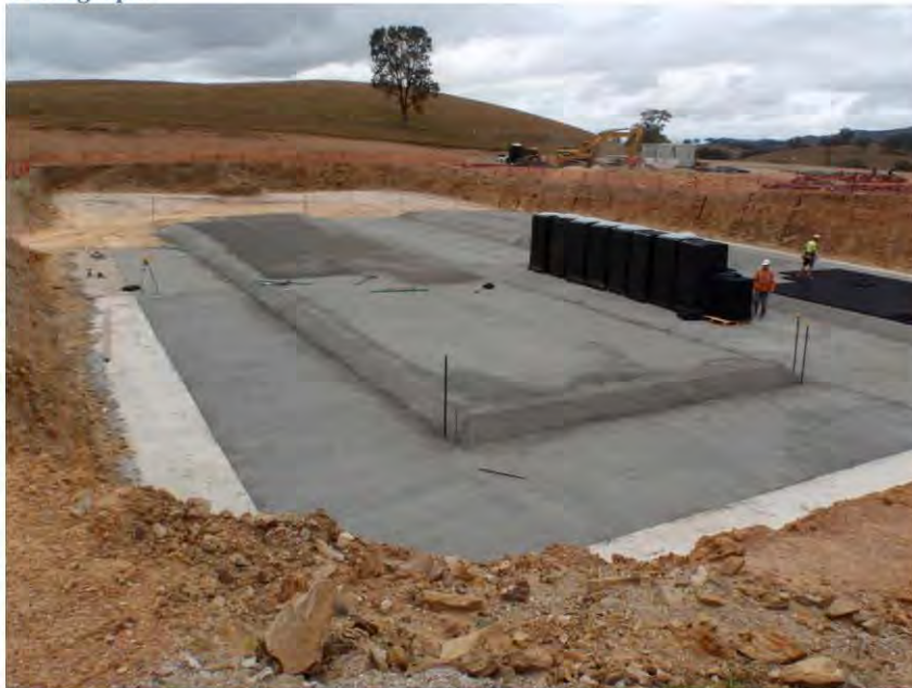
Photograph 1. Concrete blinding layer in Aeration Tank.
