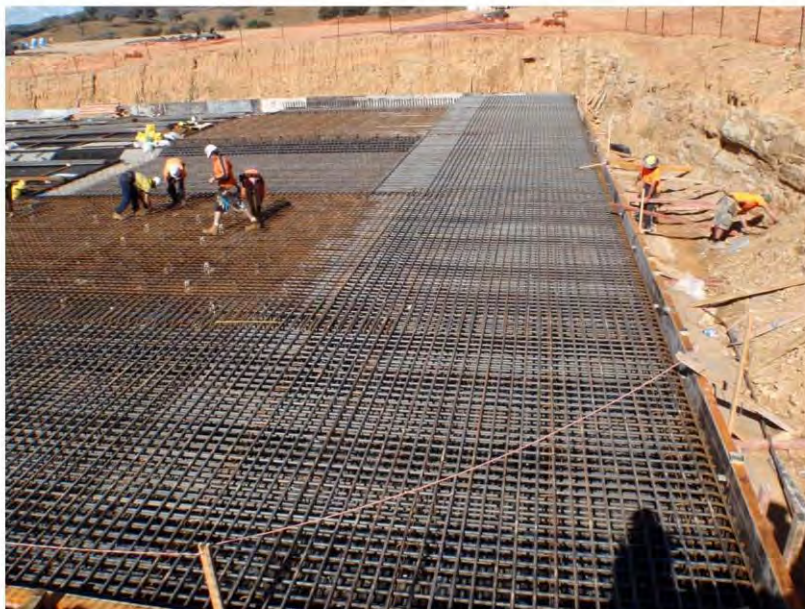
Photograph 3. Installation of steel reinforcement for Aeration Tank base.
