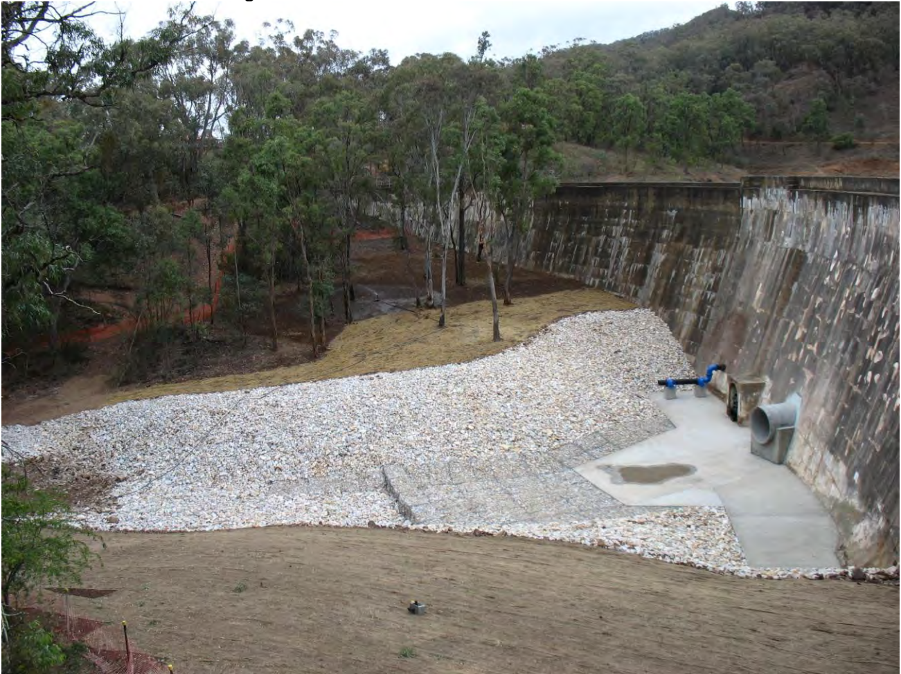
Redbank Creek Dam following construction of hole in dam wall in 2010
