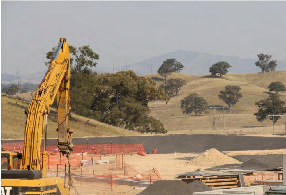
Photograph 1. Preparation of sludge lagoons prior to installation of HDPE membrane liner.
