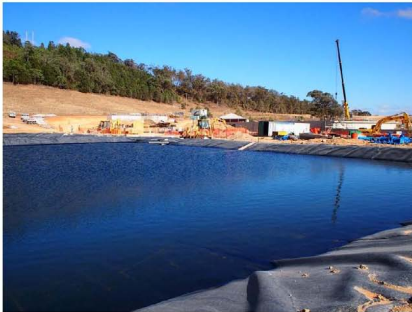
Photograph 3. Sludge Lagoon liners complete and water tested.
