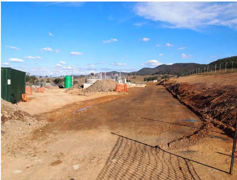
Photograph 2. Preparations for construction of site roads
