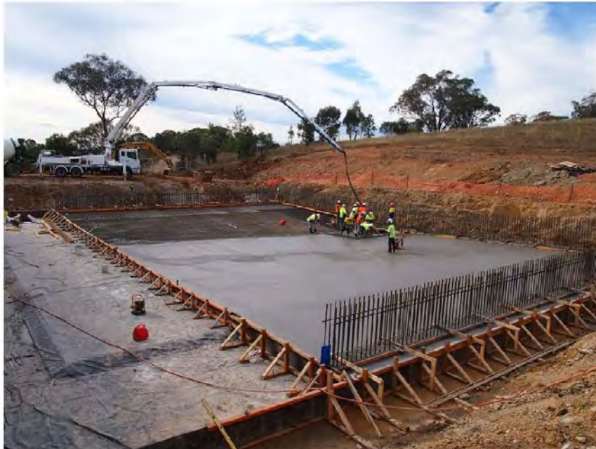
Photograph 1. Concrete pour for balance tank base.
