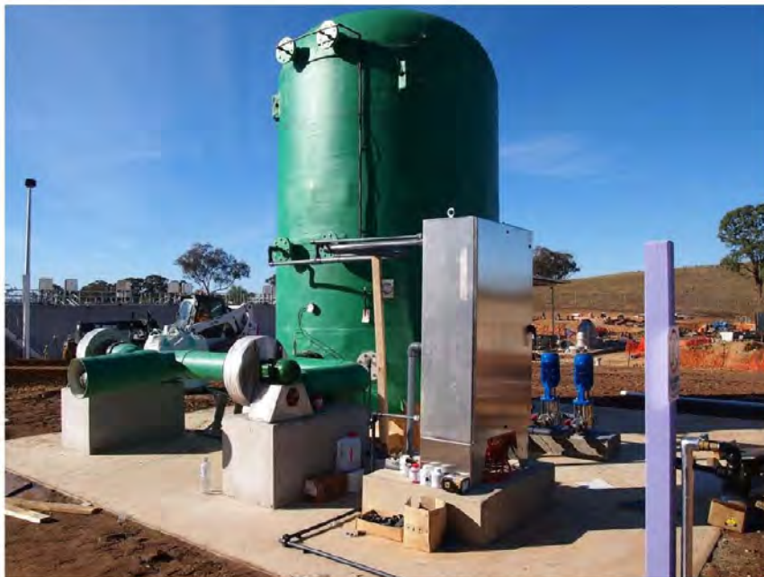
Photograph 2. Installation of controls and pipework for the odour control system
