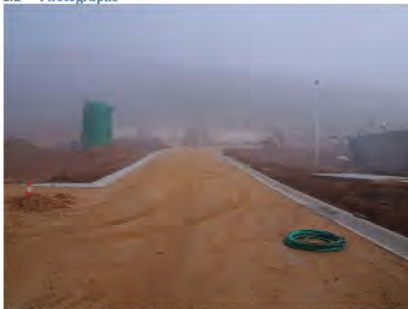
Photograph 1. Roadworks prior to sealing.
