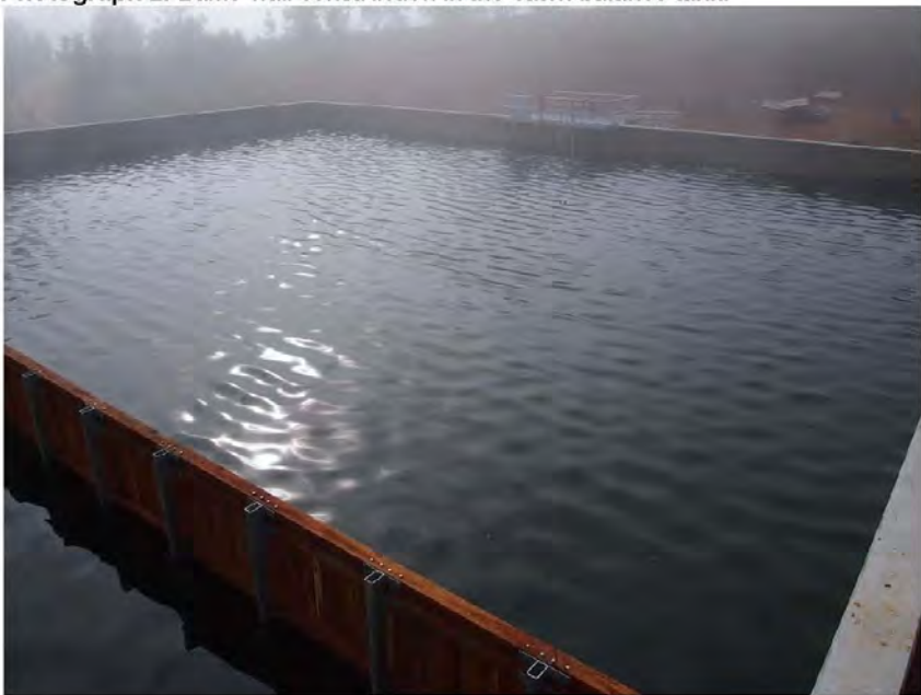
Photograph 3. Filling of catch balance tank for hydrostatic testing.
