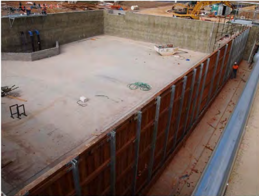
Photograph 2. Baffle wall construction in the catch balance tank.
