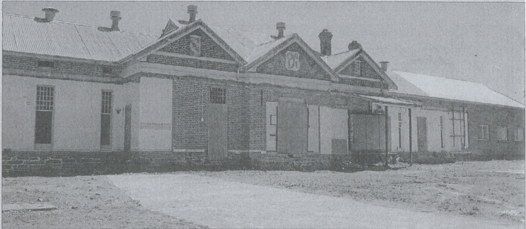
Gulgong hospital as it stands today, boarded up and stripped of its verandah.
