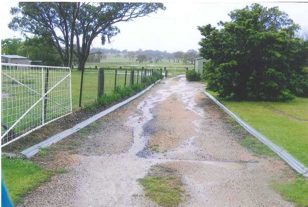
■ Figure 2-8 Stormwater running along the Driveway of 15 George Street
