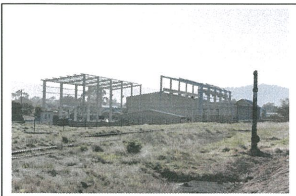
Figure 4 – Cahill Park view
