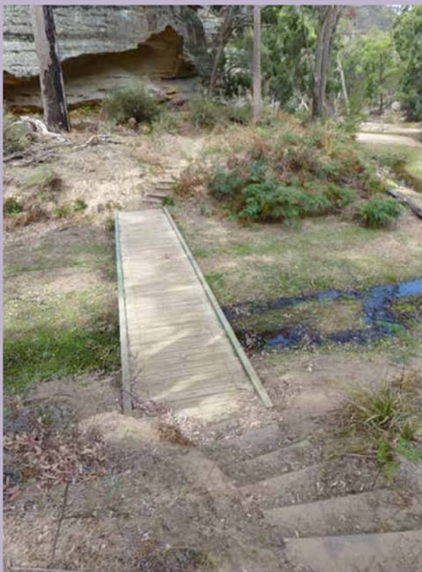
Footbridge at The Drip
