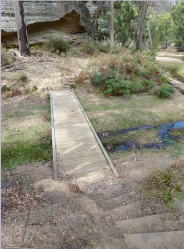
Footbridge at The Drip
