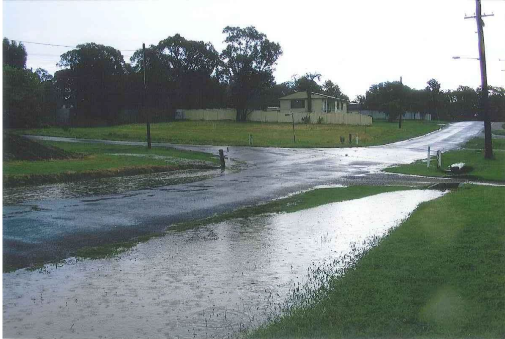
■ Figure 2-7 Stormwater impeded by culvert under the Driveway of 15 George Street
