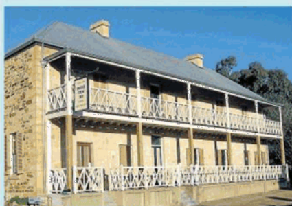
The Bridge View Hotel in Rylstone.
