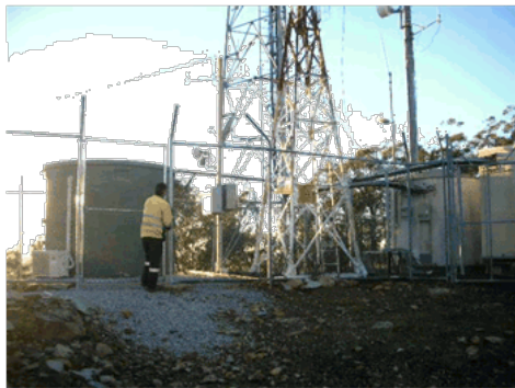
View of compound entry and converted concrete rain water tanks
