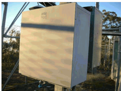
View of electrical installation
