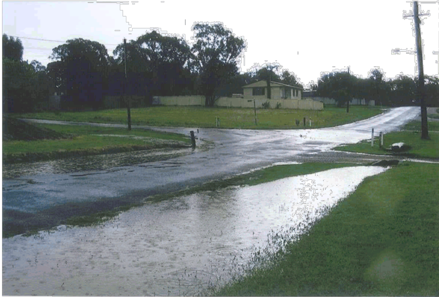
Figure 3-2 Stormwater impeded by culvert under the Driveway of 15 George Street
