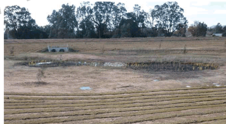
Detention basin restoration, west Mudgee.
