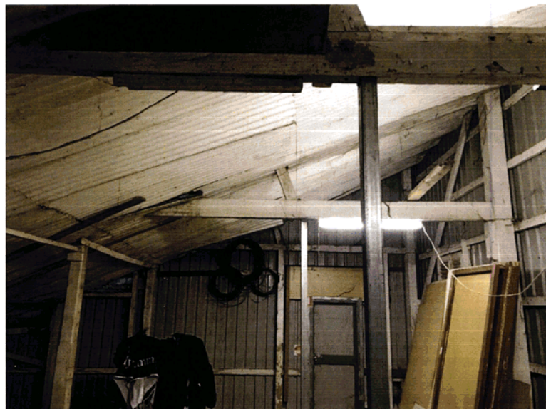
Photo No. 2 – Interim Steel Column Supports
