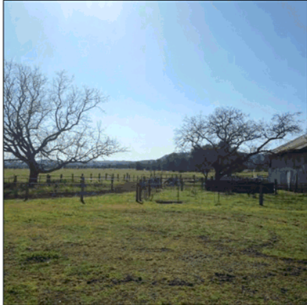
North over shearing shed and yards
