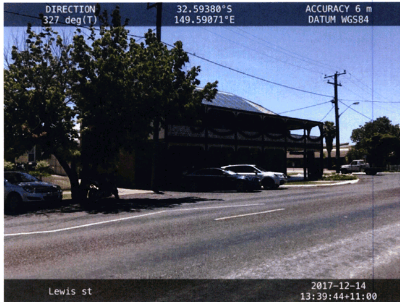
Plate 3 – Existing Oriental Hotel to the north of the site
