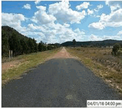
View south from the northern end
