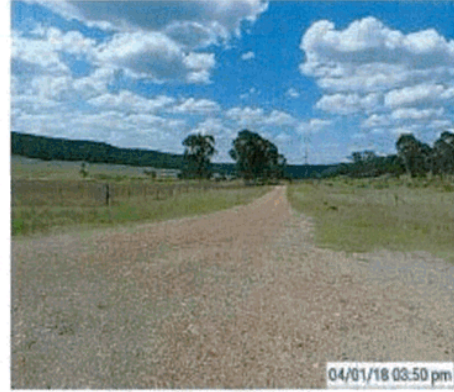
View north from the southern end
