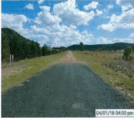
View south from the northern end
