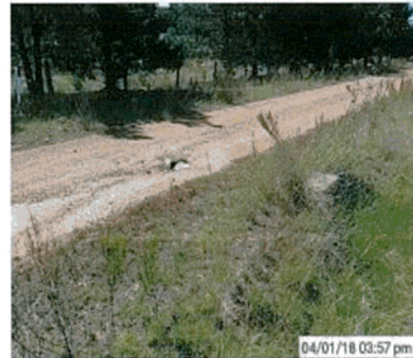
Piped Culvert traversing the Road
