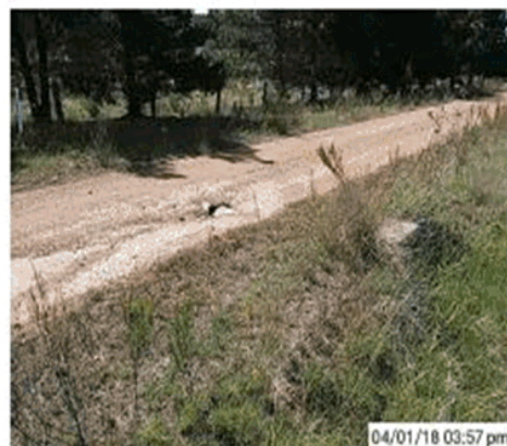
Piped Culvert traversing the Road
