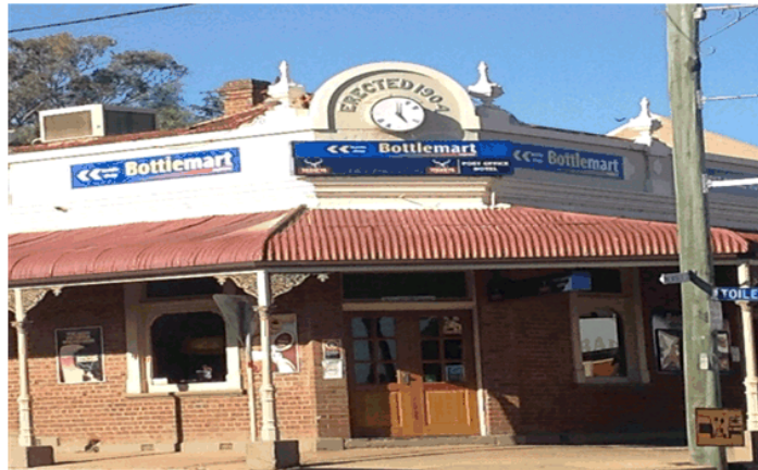
Fig. 3 Non Complying Signage
