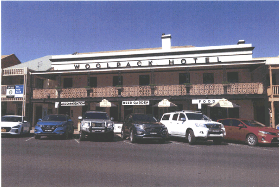
Figure 1 Woolpack Hotel façade facing Market Street BjH
