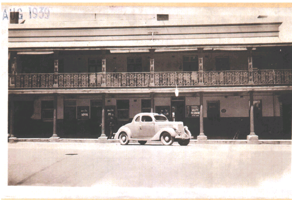
Figure 10 Club House Hotel August 1939
