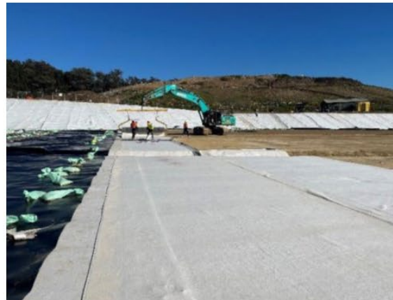
Placement of geosynthetic clay liner and HDPE liner
