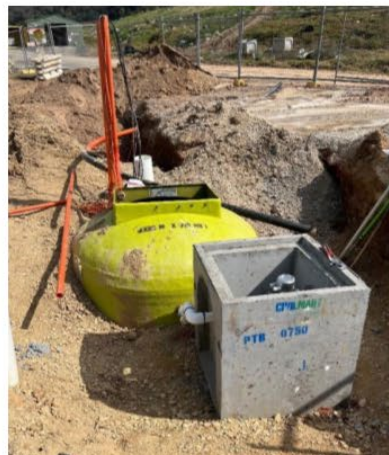
Installation of leachate pump station
