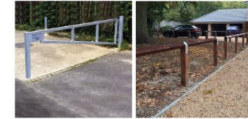
[GAT] 3700MM WIDE SWING BARRIER GATE [FEN] 600X400MM HIGH POST & RAIL FENCING
