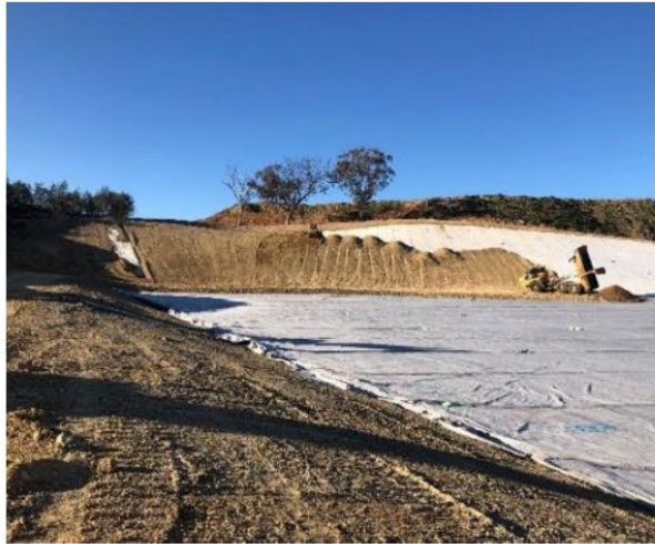
Placing of select fill
