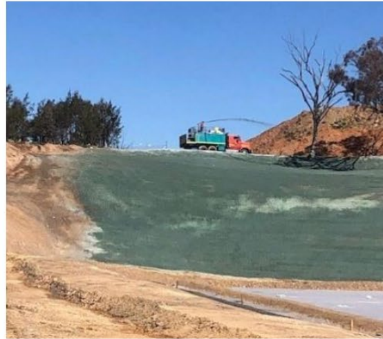
Hydro-mulching batter
