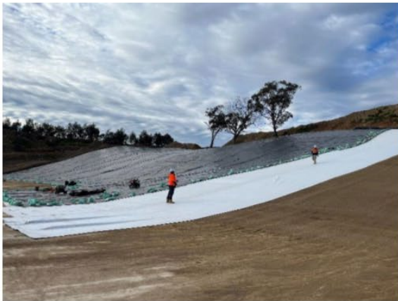
Placement of geosynthetic clay liner and HDPE liner
