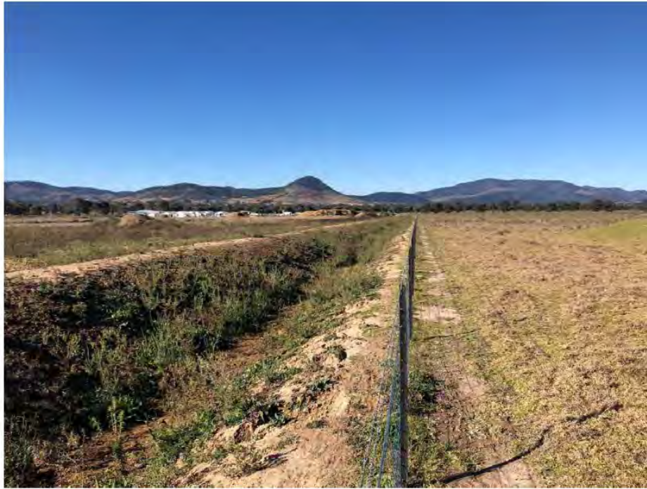
Figure 2.11: Photo I - Surface water diversion channel along outside of northern boundary fence.
