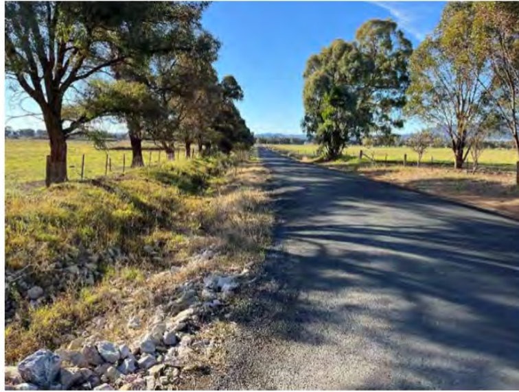
Figure 5 – Spring Flat Road, north view
