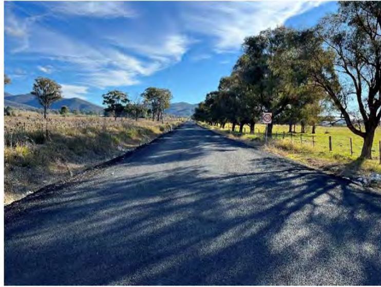
Figure 3 – Bruce Road, western view
