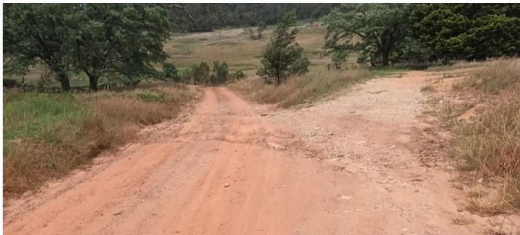
Figure 9 View of previous access way and maintained portion
