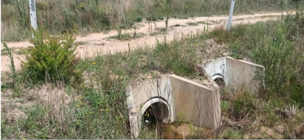
Figure 10 Culvert drains on Crown Land as discussed
