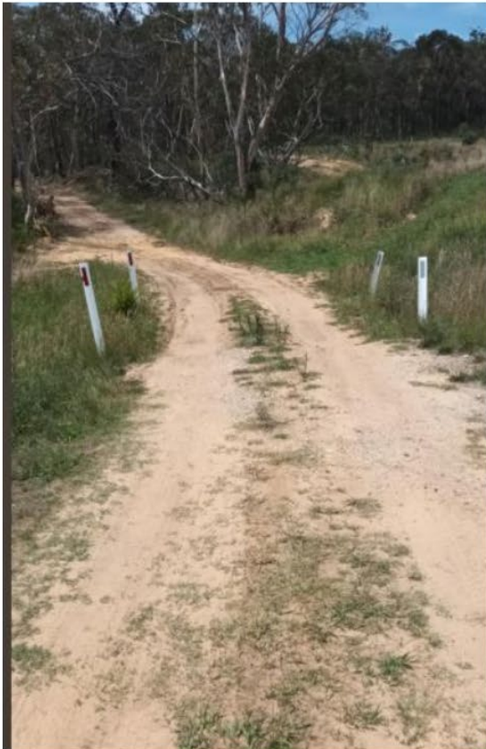
Figure 11 Culvert drain, State Forest access ahead and remainder of lots on the right in the near distance
