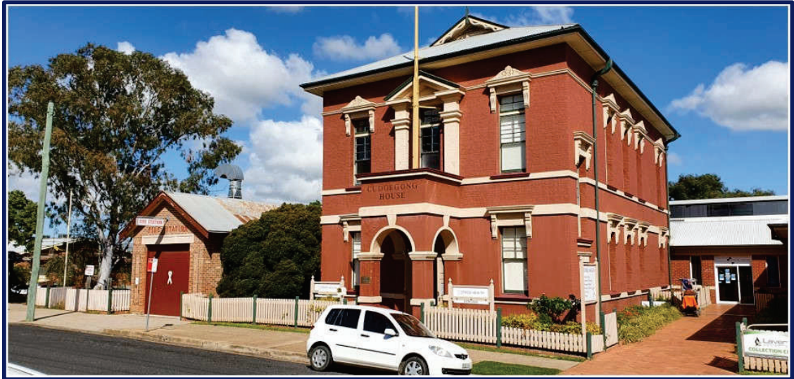
Figure 7 - Heritage Items Item I254 – Fire Station and the neighbouring I252 – Former Ulan County Council (Cudgong House)
