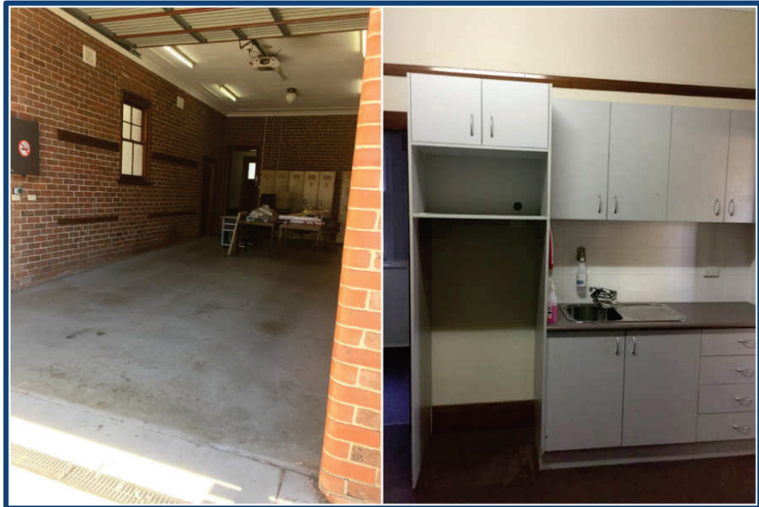
Figure 12 - Fire Station Internal Garage (left) and kitchen.
