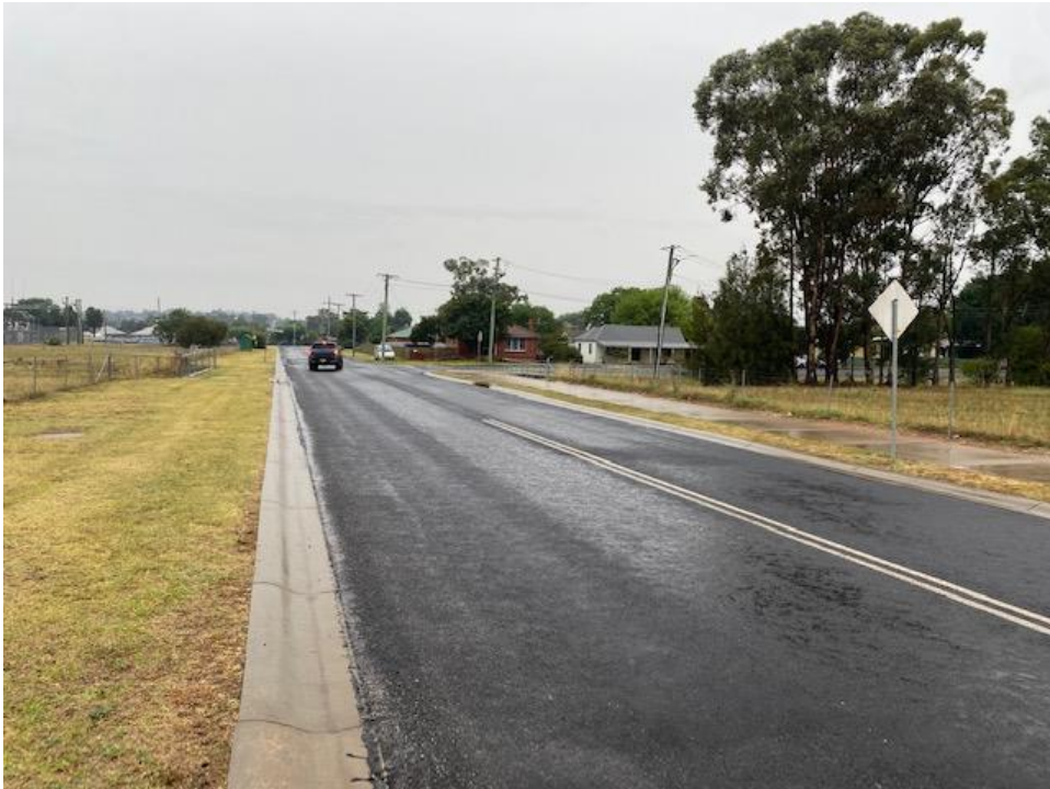
Plate 2 – View of Fairydale Lane
