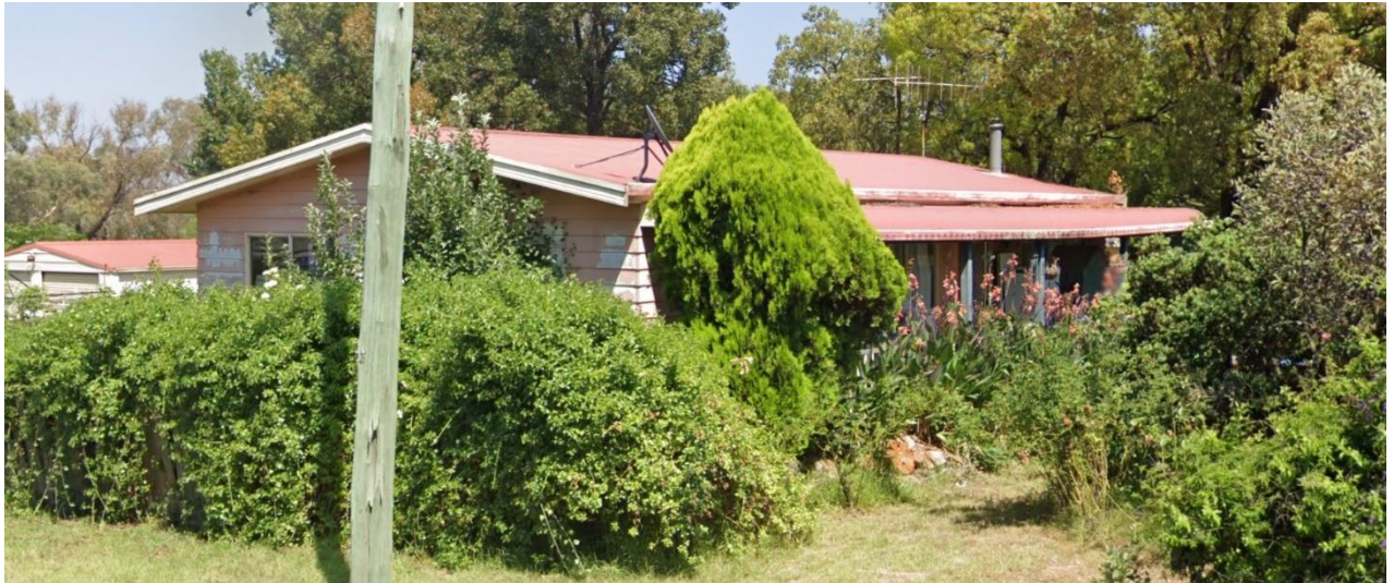
Figure 6: View of heritage-listed dwelling house at 1 Tallawang Road, as viewed from corner of Bligh Street and Tallawang Road (Source: Google Streetview)
