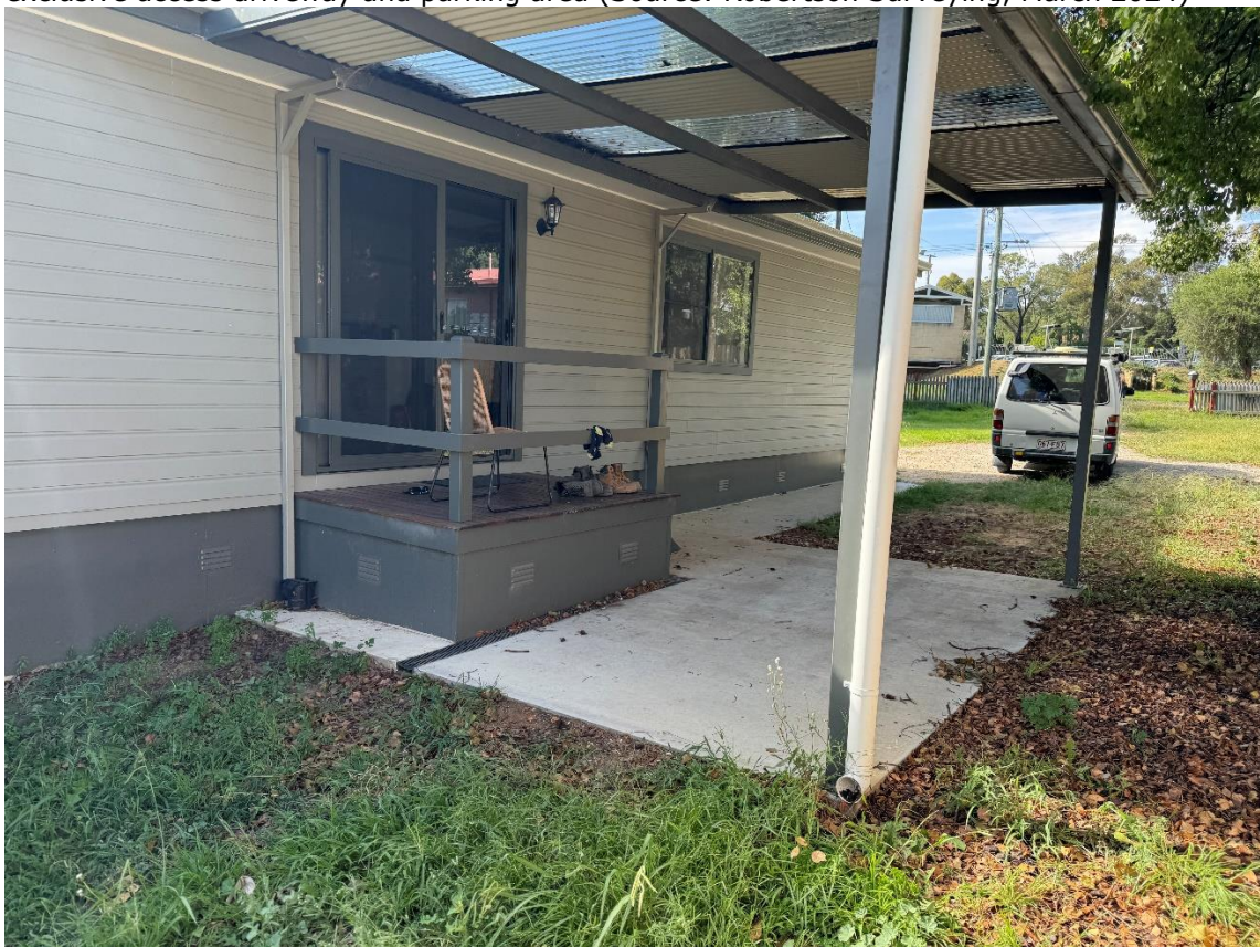
Figure 5: The existing secondary dwelling on the Site (known as 1A Tallawang Road) (Source: Robertson Surveying, March 2024)
