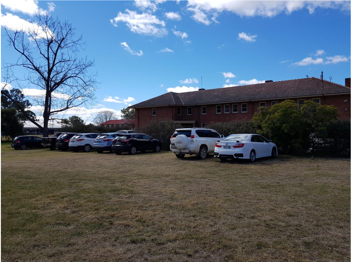
Photograph 1 - Parking on nature strip
