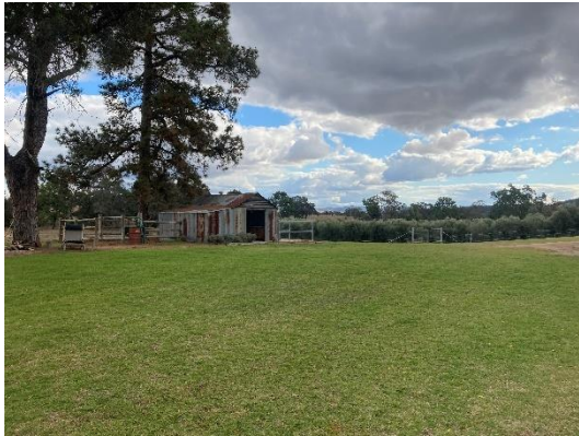
Image 7: View of shed structure on the site, olive grove in background
