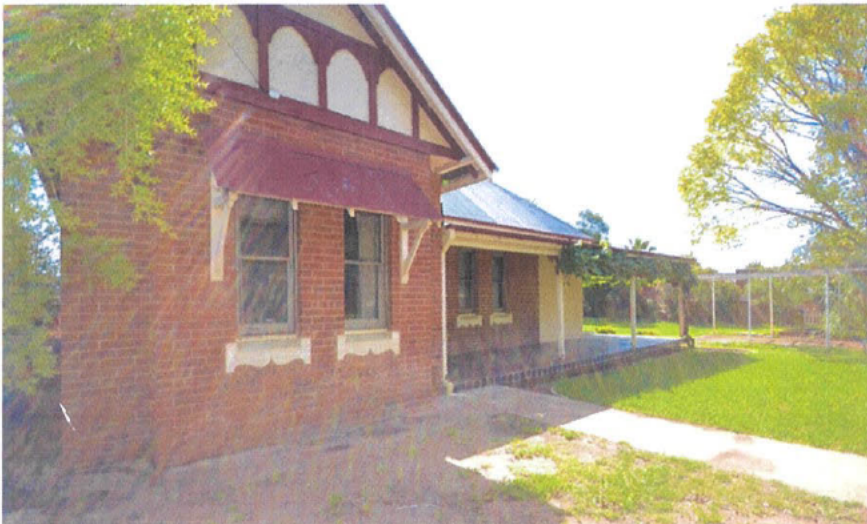
Figure 5 Facade detail facing Court Street.
