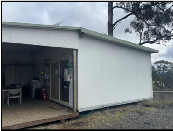
PHOTOGRAPH 3.1: Typical quarry office
