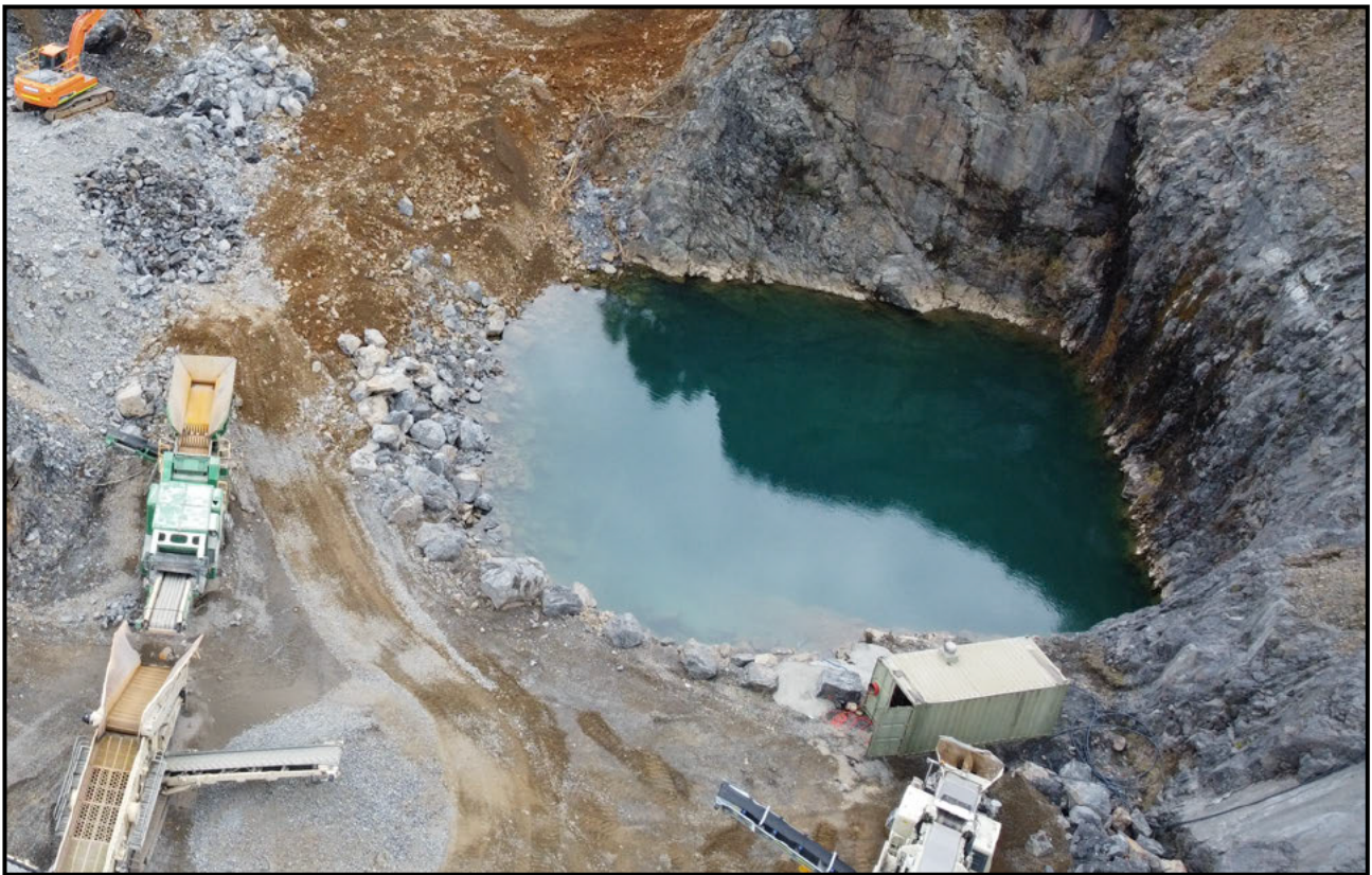
PHOTOGRAPH 3.12: Typical quarry sediment basin
