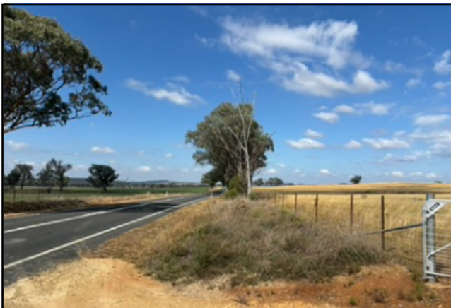
PHOTOGRAPH 7.13: View of Castlereagh Highway at entry to site looking south.
