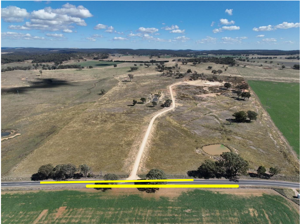
Figure 21: The indicative location of the proposed shoulder widening of the Castlereagh Hwy
