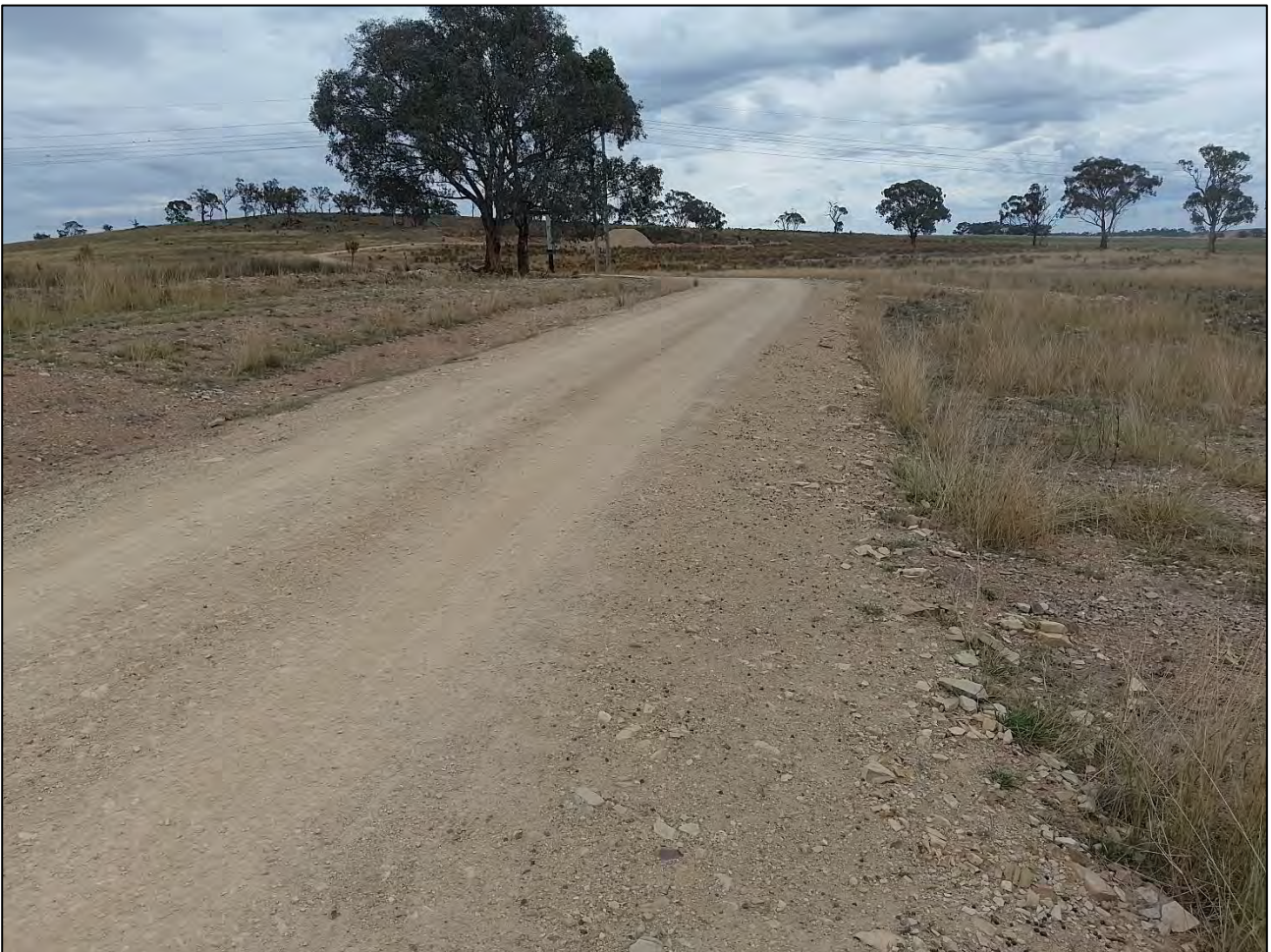
Figure 2 – View of existing access road, constructed of site won material
