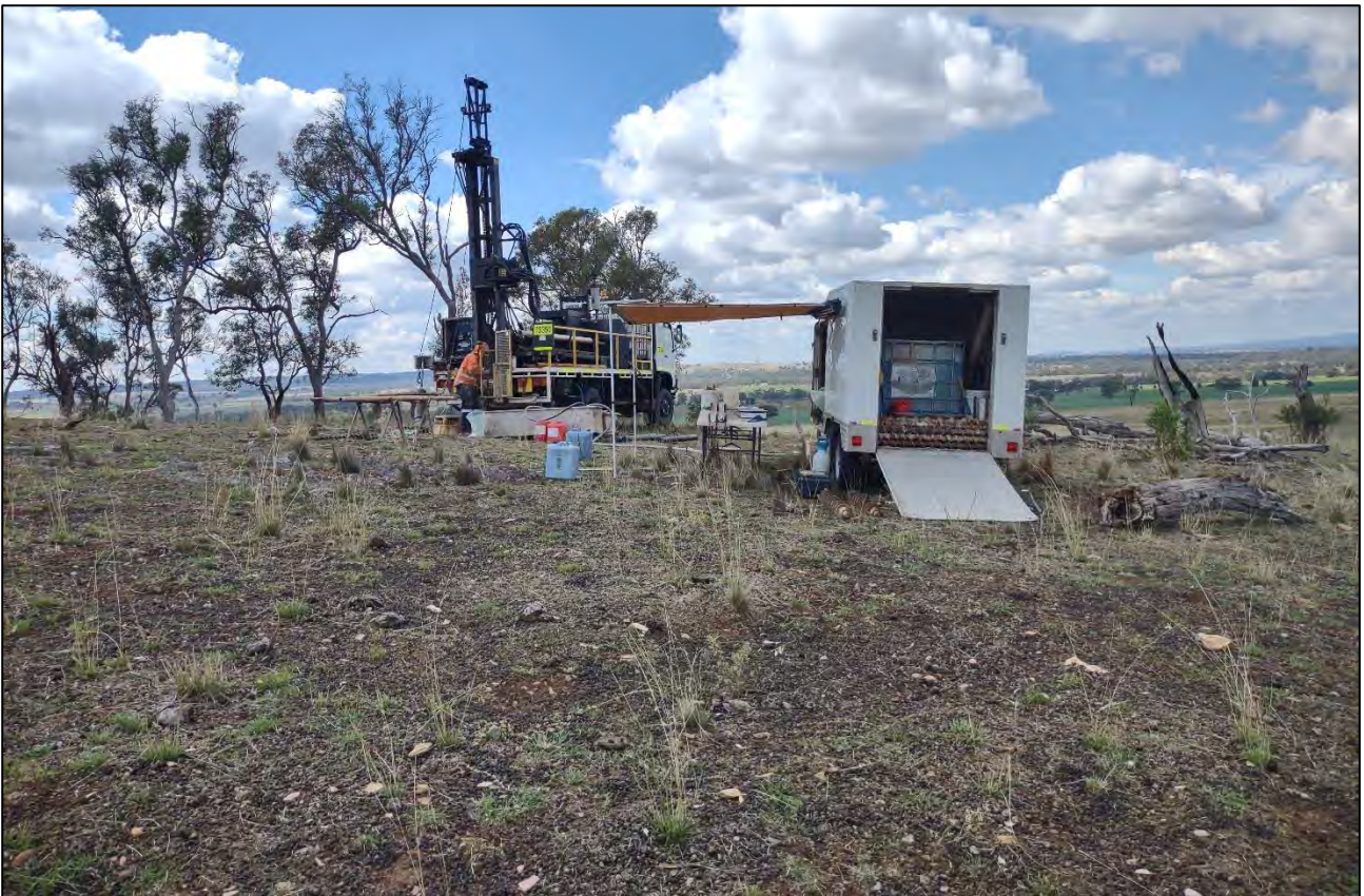
Figure 4 – View atop hill, Bore 2.
