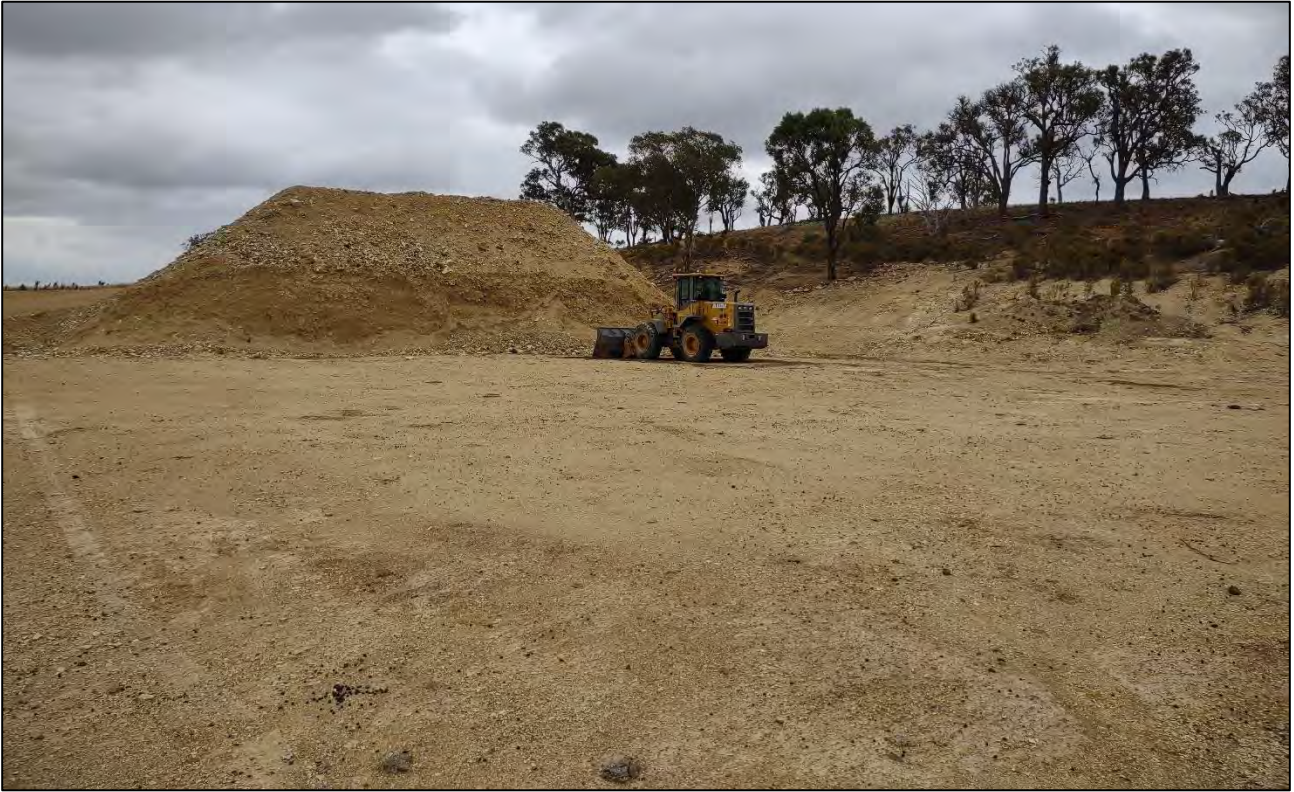
Figure 3 – View of area of existing excavation and stockpiled material, near Bore 1
