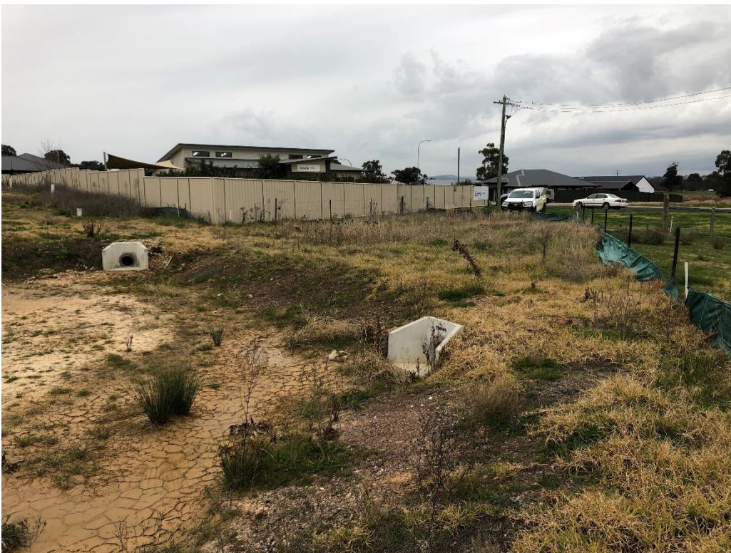
Figure 5.2: Evidence of earthworks to the south of Investigation Area
