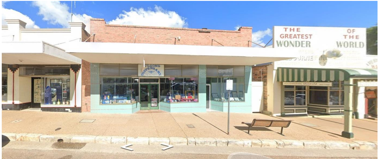
Figure 4 Typical Mayne Street parapets in Gulgong.
