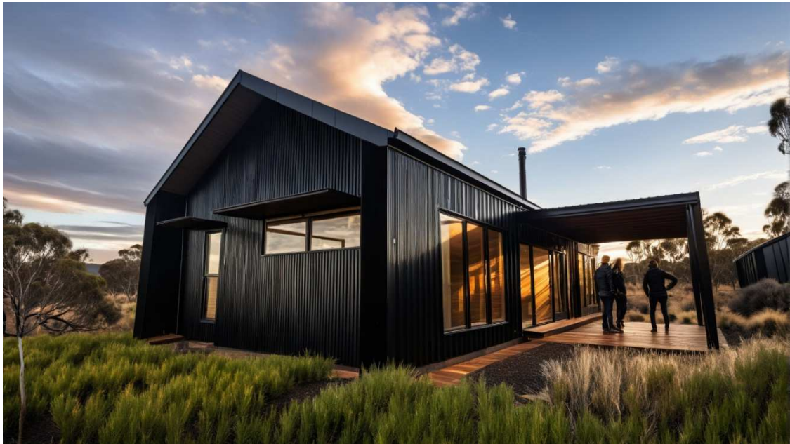
Figure 06 – Typical view of apartment. Metal cladding is complemented with charred timber cladding creating a subtle contrast. A pergola patio area adds cover/light and shadow to the façade. Windows to the north to take in good natural light and rural aspect.
