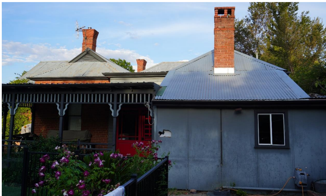
Figure 3 Rear view of house at 82 Douro Street Mudgee
