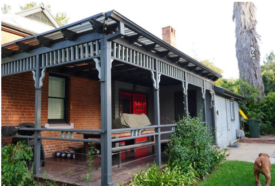
Figure 8 Rear verandah or Al Fresco area and fibro lined laundry in the distance, which will be replaced.
